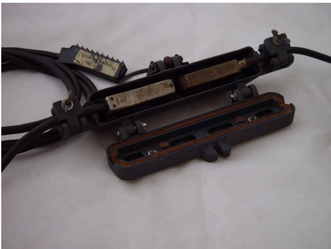
Figure 219: 30-core cable connector opened up
