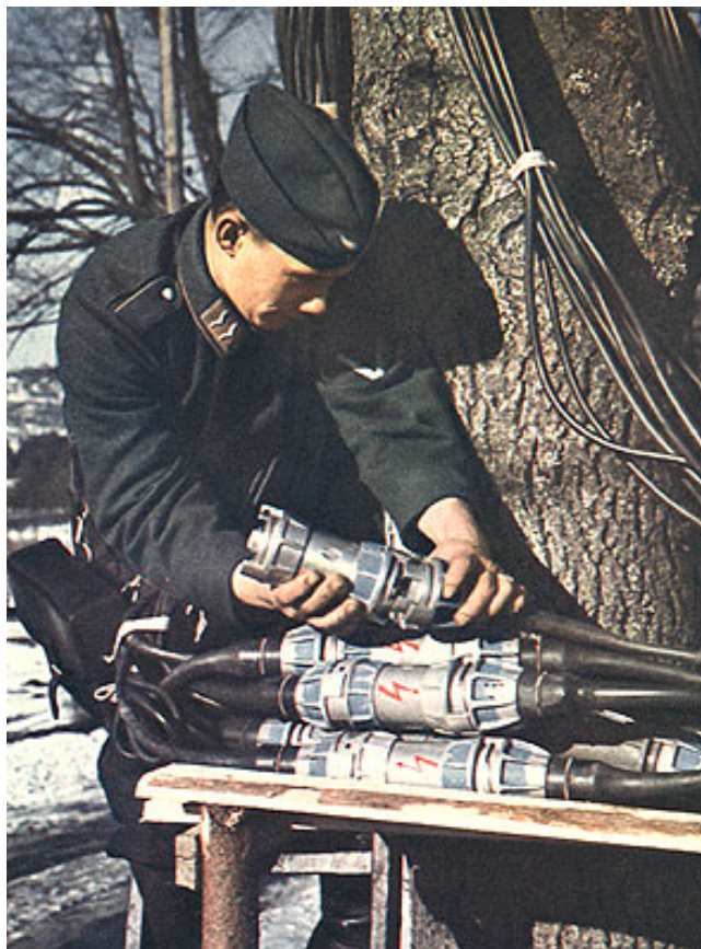
Figure 211: A Luftwaffe soldier connecting a Pupin coil to a heavy long distance field cable
