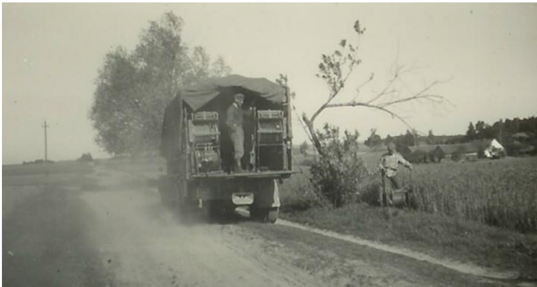
Figure 244: Schweres Feldfernkabel being built. Note the cable cart on the right of the truck
