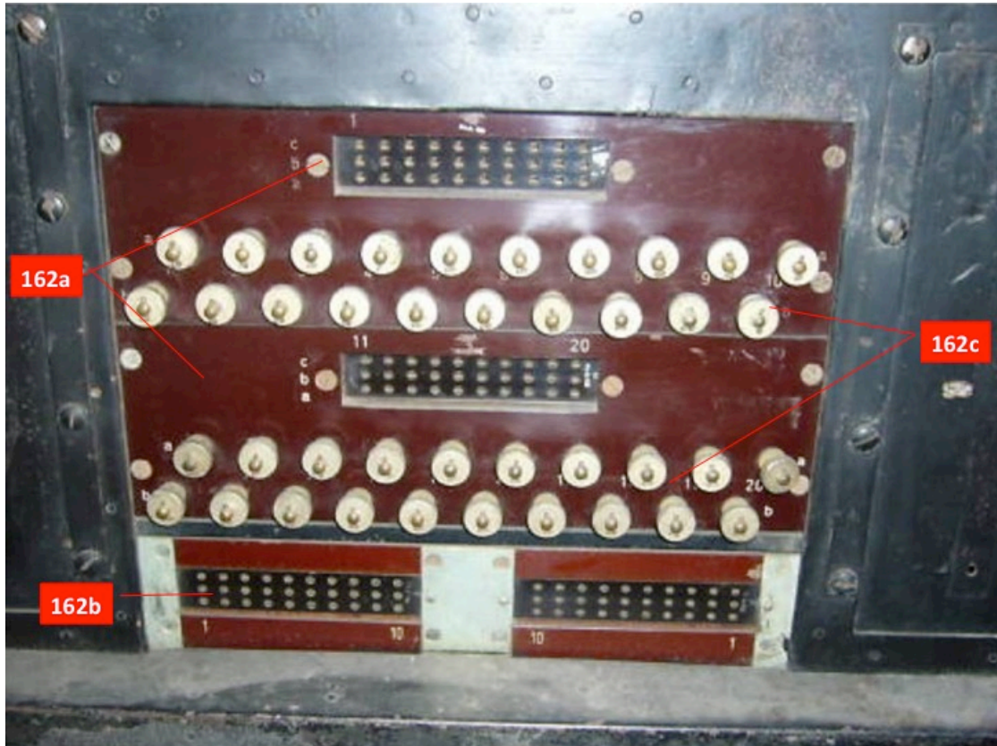
162a 30 pole sockets for remote connection of lines
