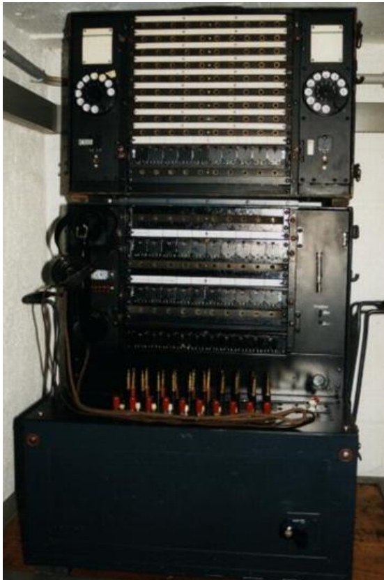
Figure 159: Enlargement unit placed on top of the exchange
