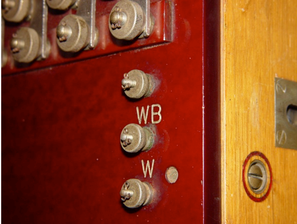
Figure 148: Terminals for an external ringer on the 10 line exchange
