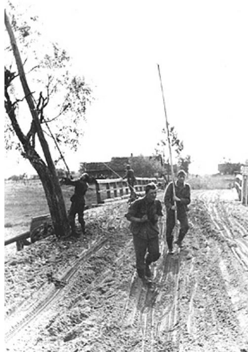
Figure 204: A light telephone troop engaged in "Geschlossene Bau" of a telephone line
